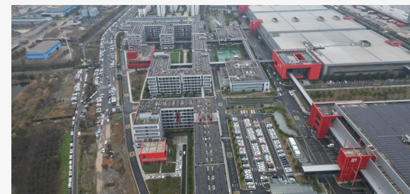
Rooftop Photovoltaic Project
